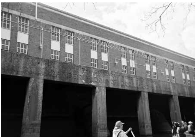
Figure 13. About thirty yards north of the southern terminus, the Racine Avenue Pumping Station (operated by the Metropolitan Water Reclamation District of Greater Chicago) pumps combined sewage wastewater from the South Side of Chicago to the MWRD's waste water treatment plant in suburban Stickney. Photograph by Laura Bryson.
